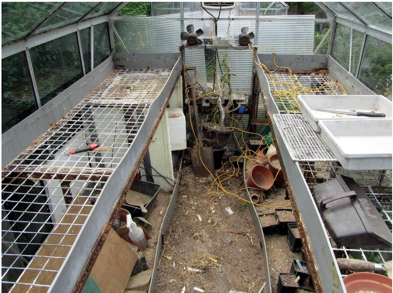
All the sand has been removed to reveal the original structure. The wire mesh was covered in polythene sheet to hold the sand – remarkably the polythene has lasted well for most of the 25 years but was pretty degraded and brittle as we removed it. We now have to cut out the old staging, remove all the clutter, sort out the old electrics then build up a new set of plunge benches which I will reveal in coming weeks.
