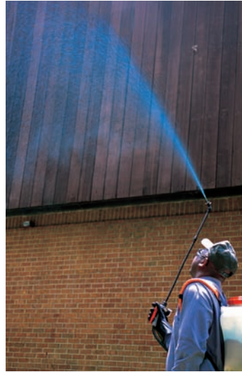
Higher spray heights achieved with narrow-angle nozzle, wand extension, and higher pressure.
