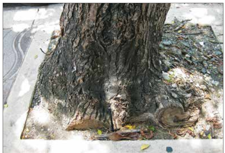
The roots of urban trees can conflict with sidewalks if they are not given sufficient growing space.
