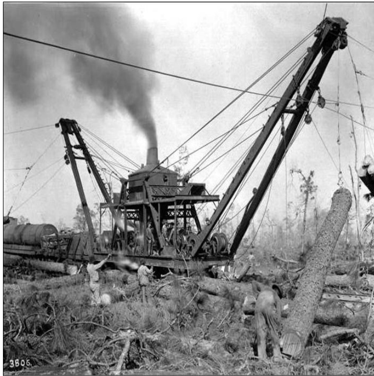
Figure 1—This massive rail-mounted Clyde skidder could harvest 40 acres of timber at one setting. Four cables could pull timber from up to 1,000 feet.
