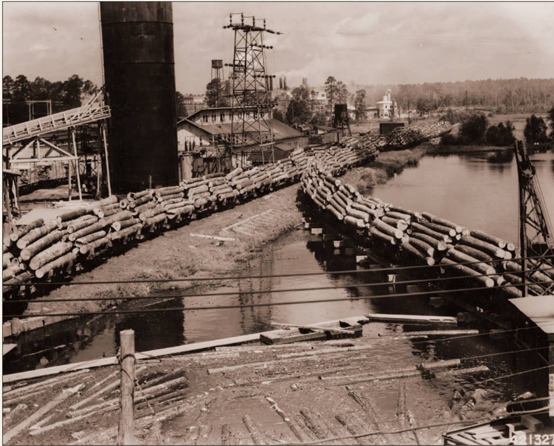
A view of the large sawmill, mill pond, and rail line of the Crossett Lumber Company indicating the large volume of lumber produced (approximately 30,000,000 feet annually) by this operation. (USDA Forest Service photo taken by Leland J. Prater circa 1942)
