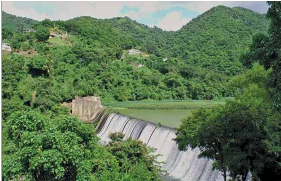
The delivery of fresh water, held here by the Rio La Plata dam, is one of the vital ecosystem services delivered by Puerto Rico's forests. (photo by Dr. Humfredo Marcano, Southern Research Station)
