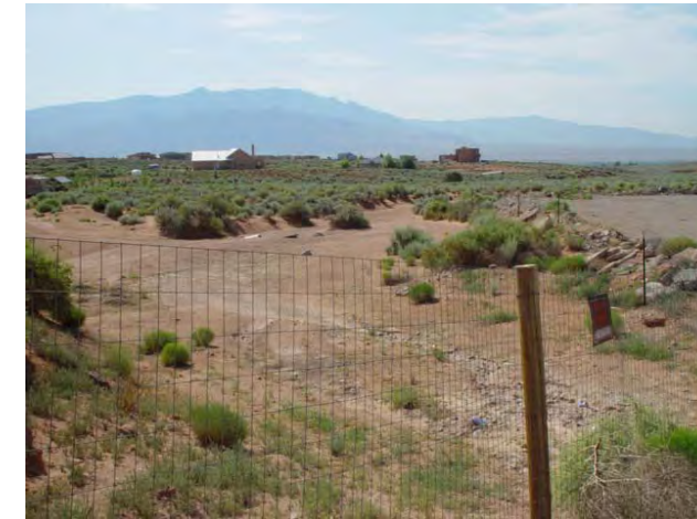
Photo 9a – Tributary BAK downstream from Iris Rd. with rubble and fence in arroyo
