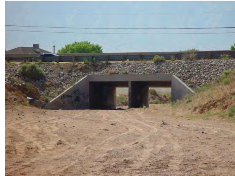
Photo 8 – Main Branch at NM 528 2 – 14' x 10' CBC
