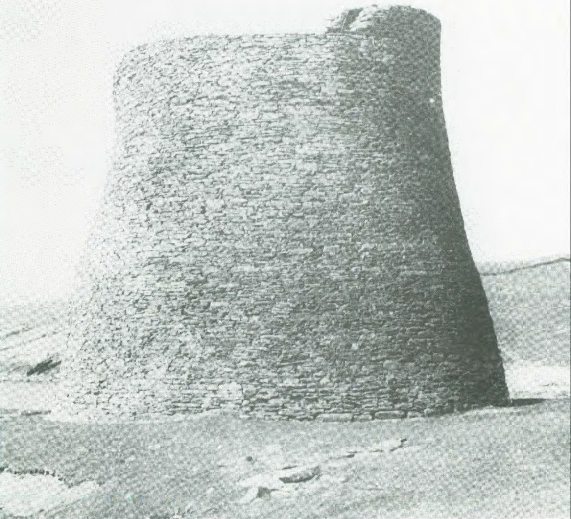
Fig. 2.1 Broch of Mousa on its small island off the east coast of Dunrossness, Shetland. This is the best preserved of all brochs and also probably the best built, the highest part of the wall still standing 43.5ft (13.3m) high. 1963.
