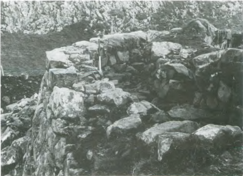
Fig. 2.21 General view of part of the galleried wall of Dun Ardtreck after excavation, showing the shallowness of the gallery and its rubble floor. Both features are the result of the hollow wall having been built on a rubble platform. 1965.
