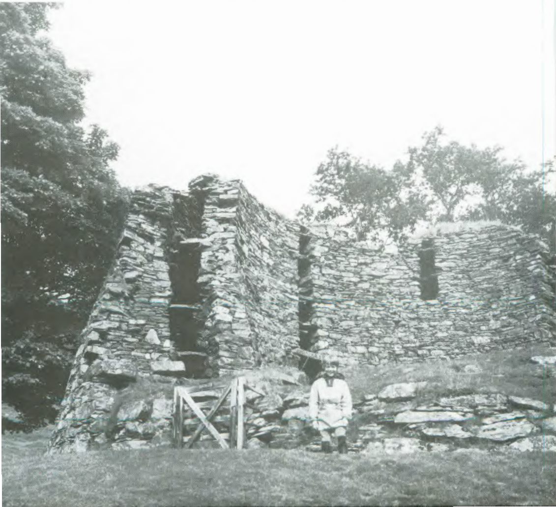
Fig. 2.2 Dun Troddan broch, Glen Beag, near Glenelg, western Inverness-shire, 1974. This has a solid base like its neighbour Dun Telve and both are more typical of the brochs of the far north than of the west. The hollow, double wall is clearly visible in cross-section on the left, as are two vertical rows of windows or voids in the interior wallface.
