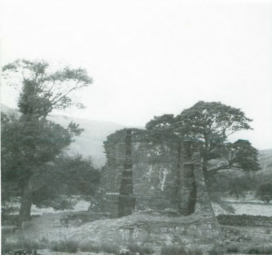
Fig. 2.3 Dun Telve broch, Glen Beag, near Glenelg, western Inverness-shire, 1963. This solid-based broch with its high, hollow or galleried wall was almost as well preserved as Mousa when Alexander Gordon saw it in about 1720. Shortly afterwards it was badly damaged by a contractor, presumably he who was building the barracks at Glenelg in 1722.
