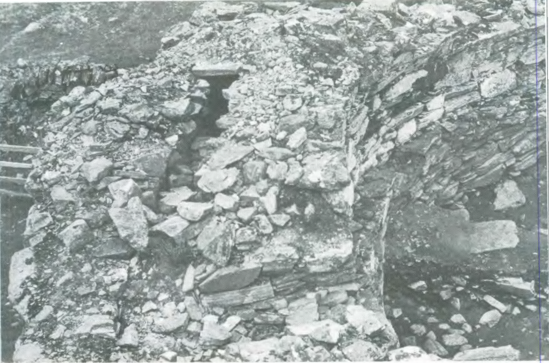
Fig. 2.25 Dun an Ruigh Ruaidh. General view of the semibroch in 1978 after excavation. In the foreground is the raised doorway from the interior to the upper part of the intramural stair. It was reached from the raised wooden floor resting on the scarcement visible on the inner face. The remaining steps have been re-buried but the flight ran up above the upper gallery visible in the middle of the wall, which therefore ended blind behind the stair.
