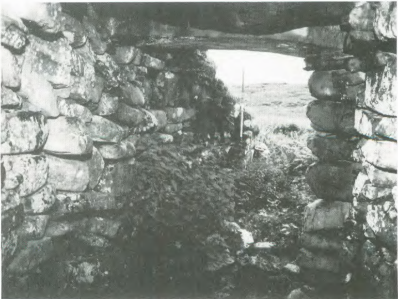
Fig. 2.8 The entrance passage of Dun Ringill semibroch, looking out, 1988. The original Iron Age lintels have been re-set over the Medieval inward extension of the passage, the junction of which with the older wall can be seen on the right, forming a door-check. The pole is at one of the door-checks of the unroofed Iron Age passage.
