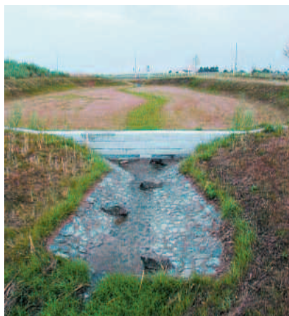
Retentionsmulde in Kalbach
