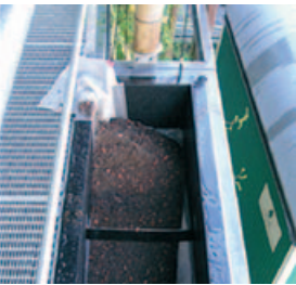
Planters with substrate on the façade
