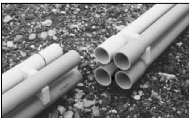
2. A thin coating of Carlon Quick Set Cement should be applied to the inside surface of the sockets lightly enough to prevent the formation of a bead of cement at the interior shoulder of the sockets. Then, apply in the same manner to the spigot ends of the conduits to the depth of the socket.
