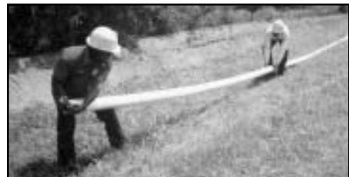
**1.** Distribute Multi-gard sections along the sides of the trench with male ends pointing towards starting vault entrance.
