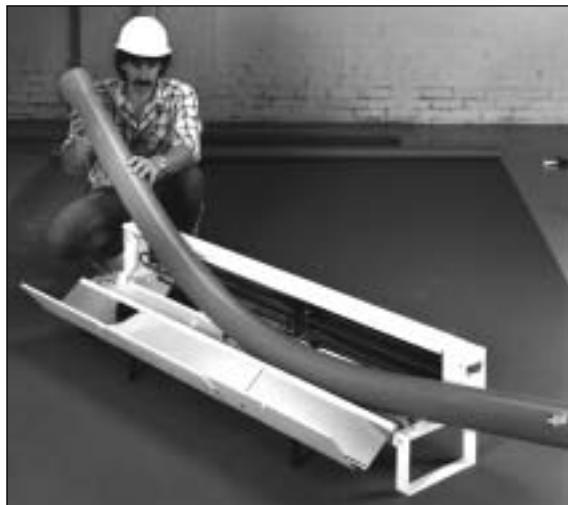
Minimum practice is required to master the three steps in bending nonmetallic conduits and ducts.
