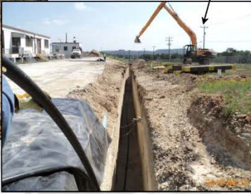
Gravel added and leveled. Injection lines installed.
