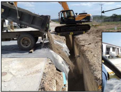
Gravel added and leveled. Injection lines installed.
