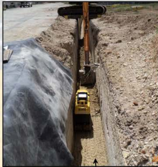
Clay layer added and compacted.
