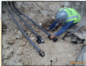
Injection headers installed.
