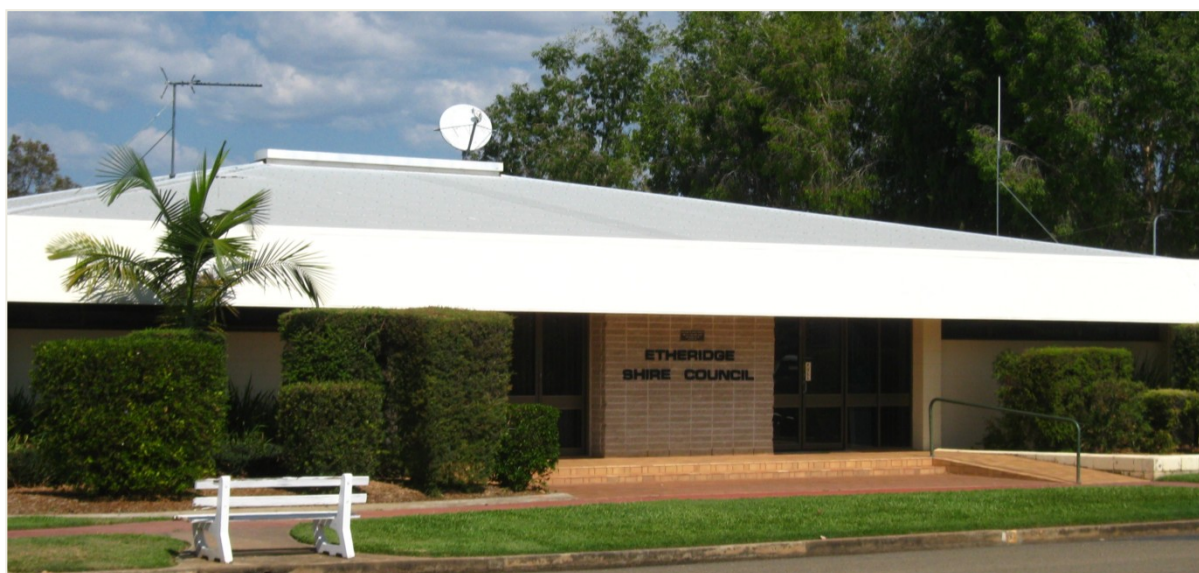
Figure 22 - Etheridge Shire Council
