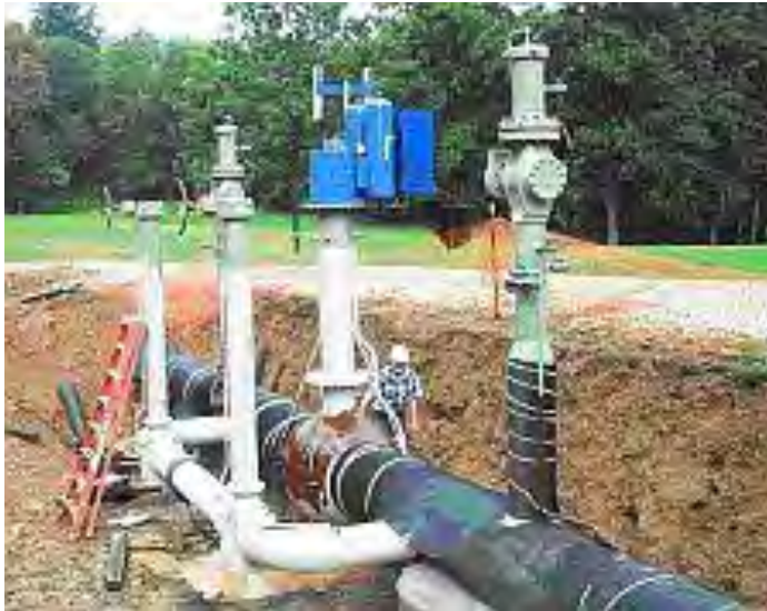
Figure 8: Typical MLV Assembly
