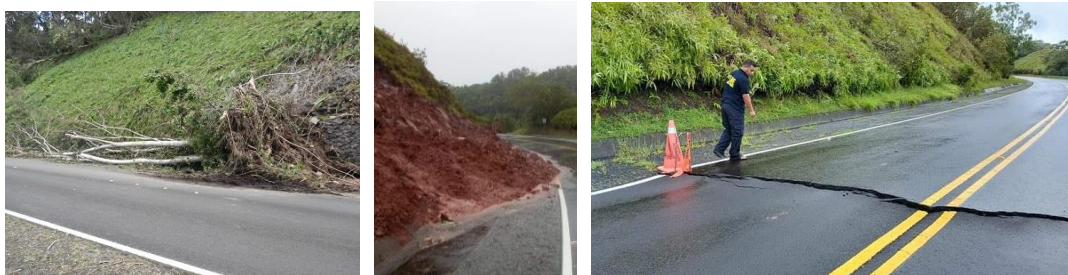
Figure 1.12 Slope failure in Ngeremlengui (left) and Ngchesar (center), and road damage in Ngardmau (right) after Super Typhoon Surigae April 2021. Slope failure sites are priority sites for stabilization of slopes to prevent forest loss.
