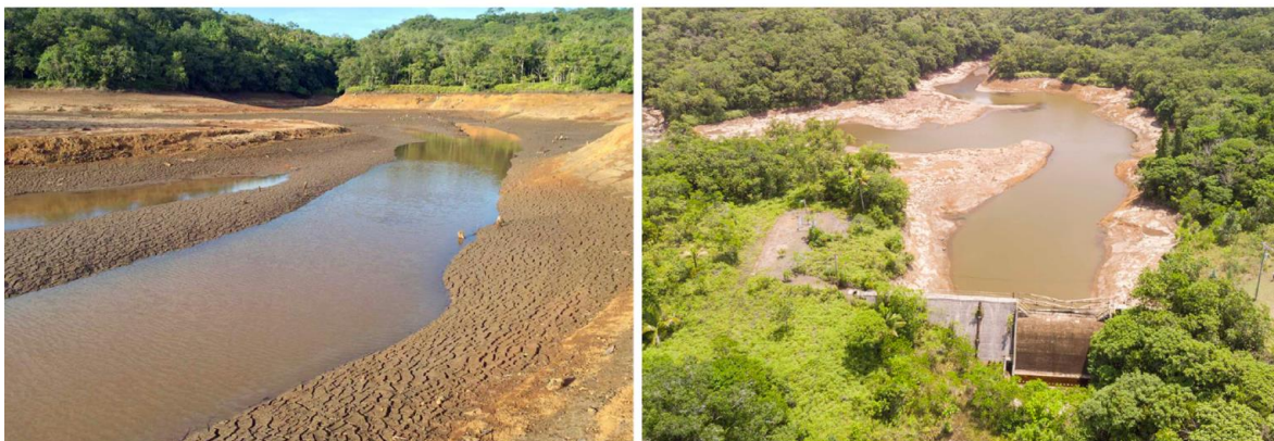
Ngerimel Dam - Mar 2016 (Photo by: OTV production).
