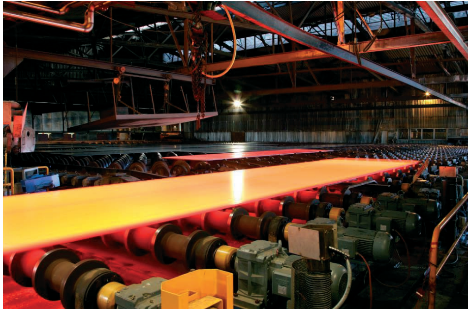
Siemens VAI and DanSteel consider that the plate mill upgrade project has been a success and demonstrates the benefits of co-operative working
