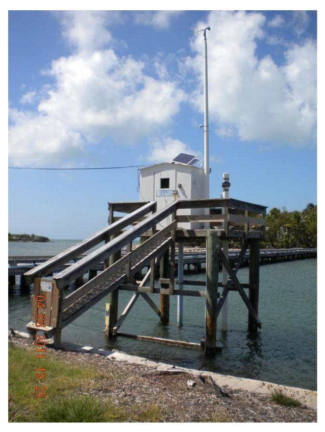
**Figure 4: NOAA Tide Gauge at Vaca Key, FL**. Image obtained from <a href="http://tidesandcurrents.noaa.gov/stationphotos.html?id=8723970#">http://tidesandcurrents.noaa.gov/stationphotos.html?id=8723970#</a>, accessed November 19, 2015.
