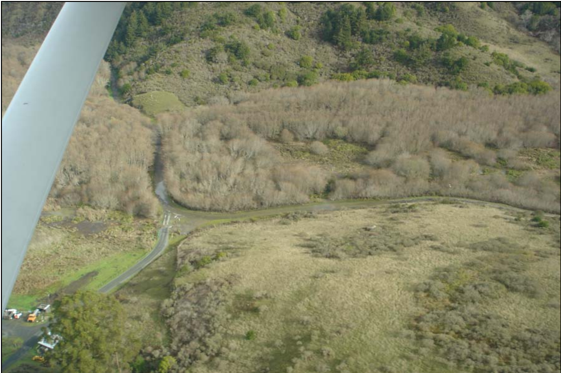
Figure 2. Aerial view of Second Bridge crossing after high flows on January 28, 2008. Note ponded water at culvert locations and southern approach.
