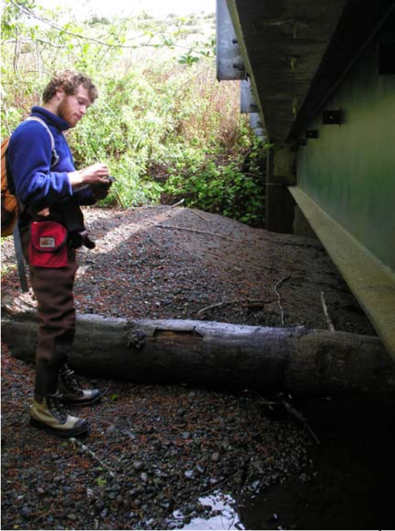
S1-C: Channel directly downstream of 3 rd bridge.
