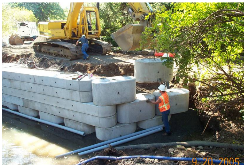
Precast concrete bridge abutments
