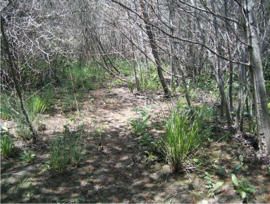
Photo 13: Abandoned segment of historic flood control channel
