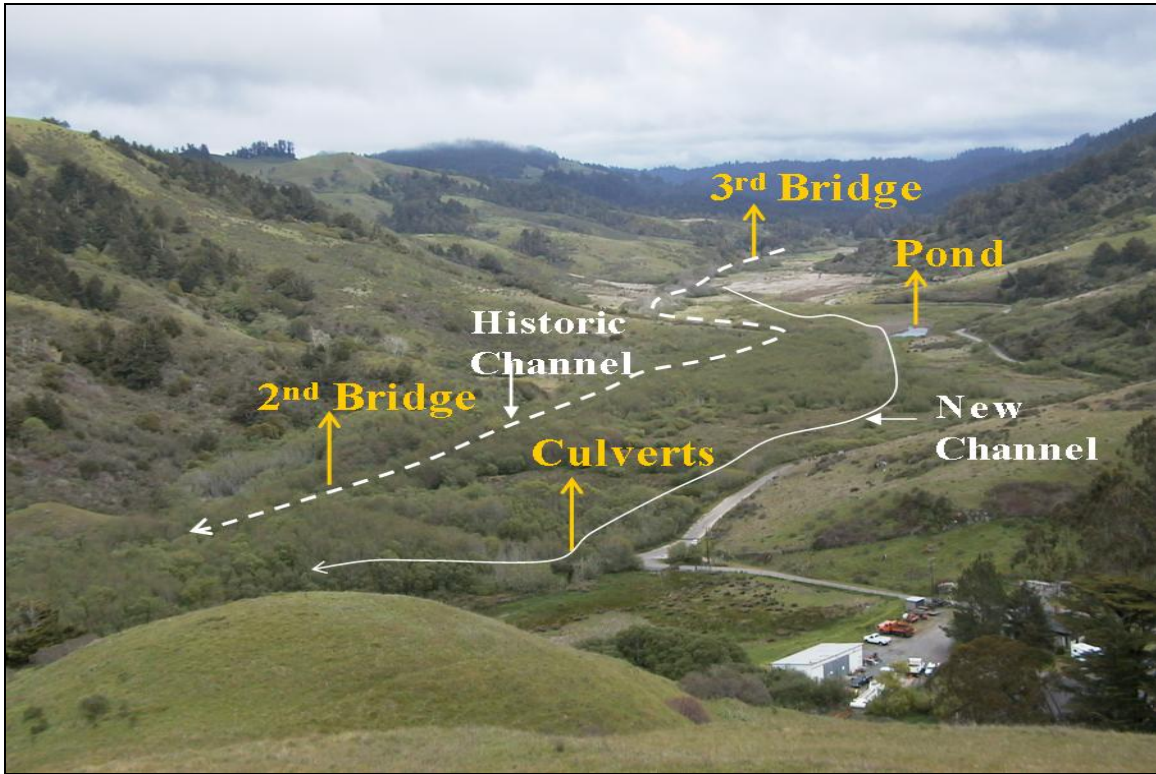
Figure 1. Lower Willow Creek with features shown that relate to this project (photo looking up the watershed).
