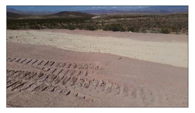
**Figure 3.** Completed GRF and RIP cells at Lime Hill. Bulldozer tracks were smoothed by raking at all sites.
