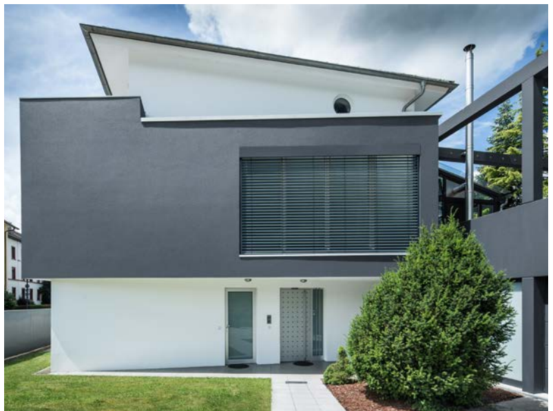
StoColor Dryonic®, Stolit® K 2, residential building in the district of Lörrach, Germany
