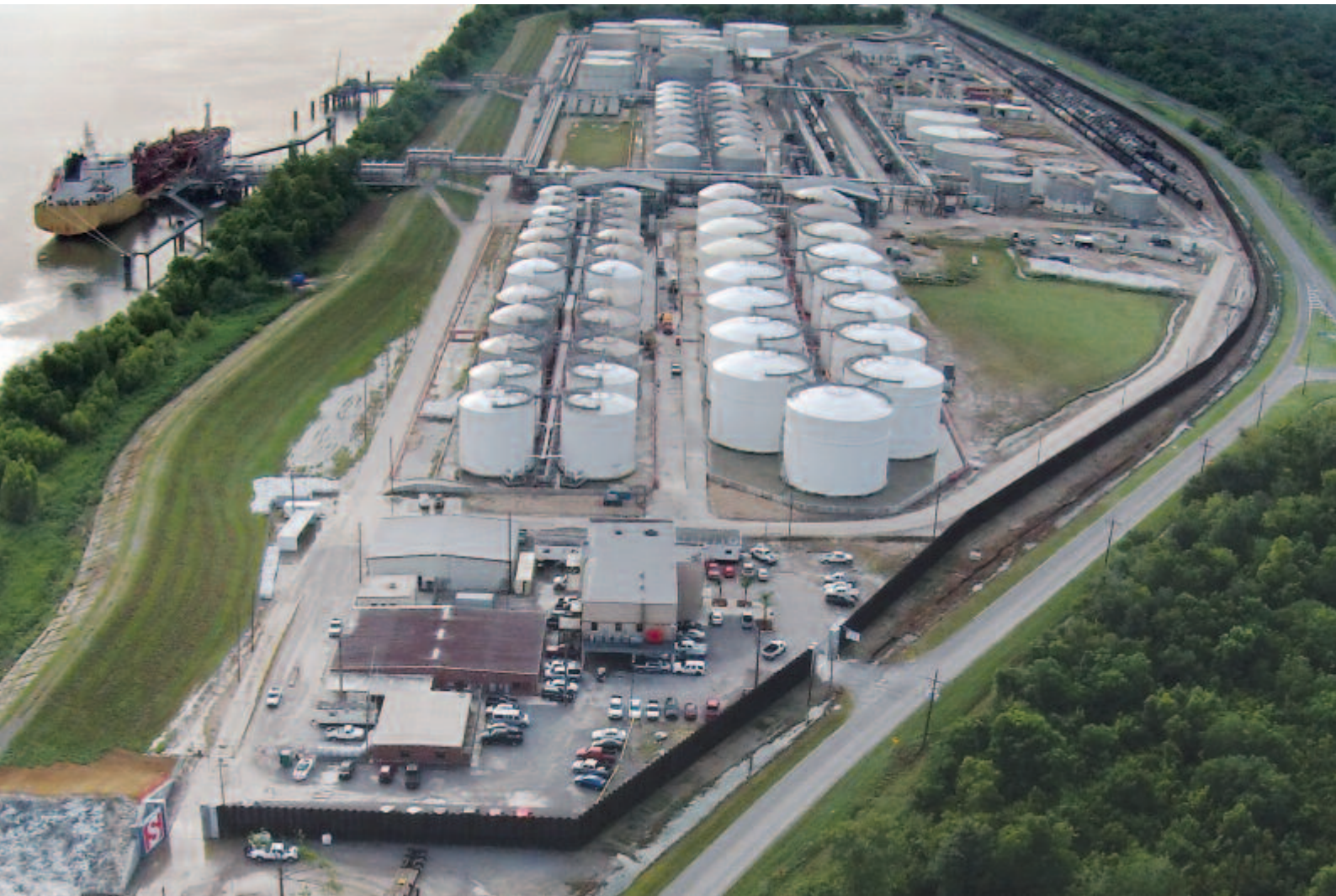
Completed in 2014, the 4,600 ft wall protects Stolthaven New Orleans from floods.
