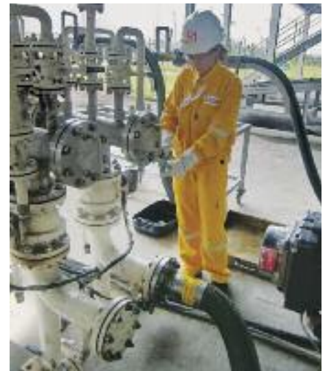
Zhang Jun carrying out operations fieldwork at the truck loading bay.
