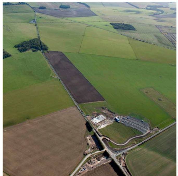
Stonehenge Visitor Centre under construction following Environmental Impact Assessment
