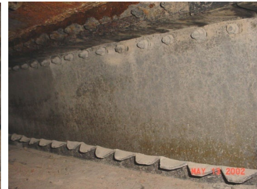
Lower Ash Hopper Damaged Seal (Due to In-Adequate Water Flow & Ash Build Up)
