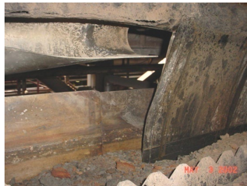
Lower Ash Hopper Damaged Seal (Due to In-Adequate Water Flow & Ash Build Up)
