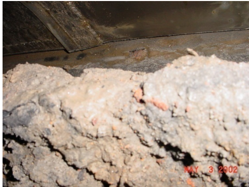
Lower Ash Hopper Damaged Seal (Due to In-Adequate Water Flow & Ash Build Up)
