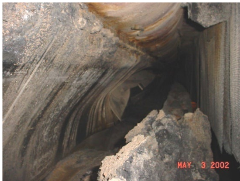
Lower Ash Hopper Damaged Seal (Due to In-Adequate Water Flow & Ash Build Up)
