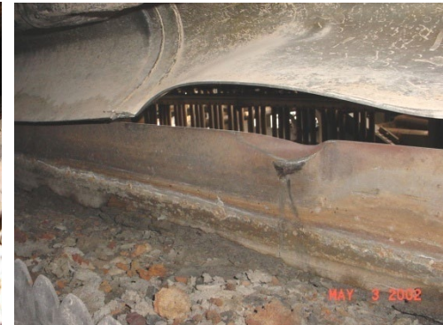
Lower Ash Hopper Damaged Seal (Due to In-Adequate Water Flow & Ash Build Up)
