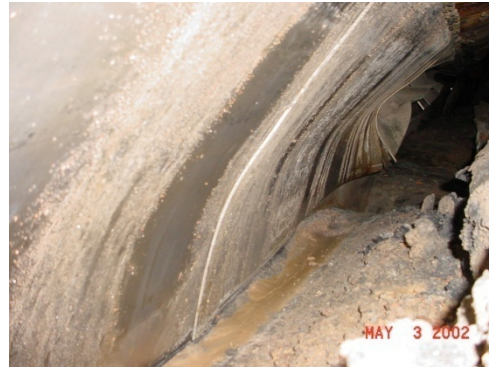
Lower Ash Hopper Damaged Seal (Due to In-Adequate Water Flow & Ash Build Up)
