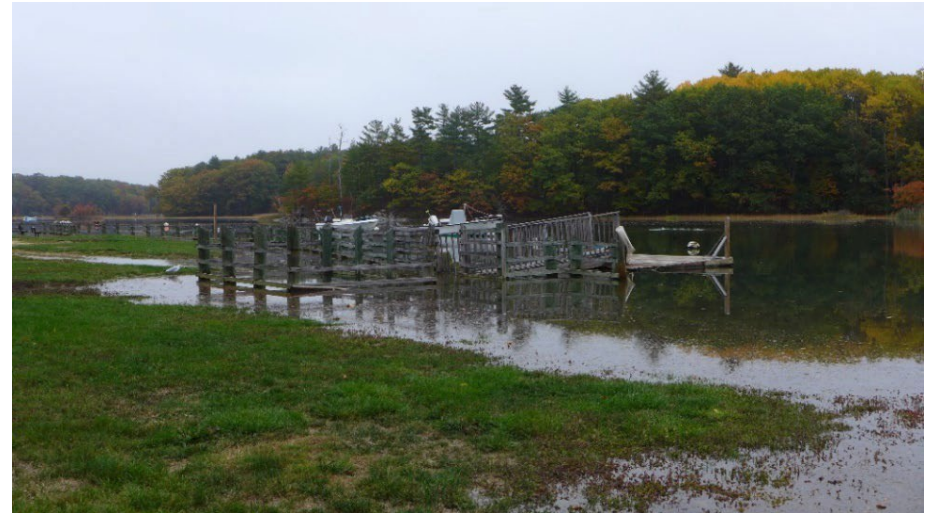
Coastal Flooding at Town Landing during 2017 King Tide Event (Photo Credit: Strafford Regional Planning Commission)
