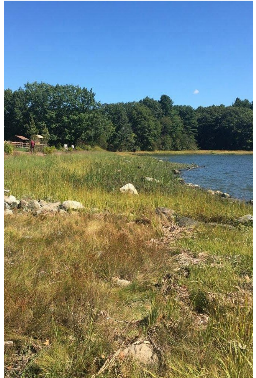
Living Shoreline Installation at Wagon Hill on Great Bay (Photo Credit: NHDES)
