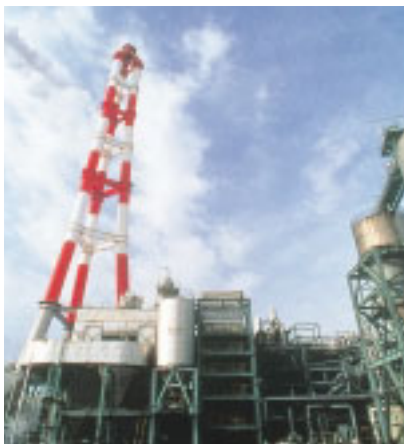
Proprietary technology used for denitrification
