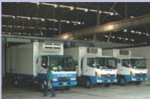
The logistics center in Urayasu boasts a complete temperature control system with freezing, chilled and room temperature settings.
