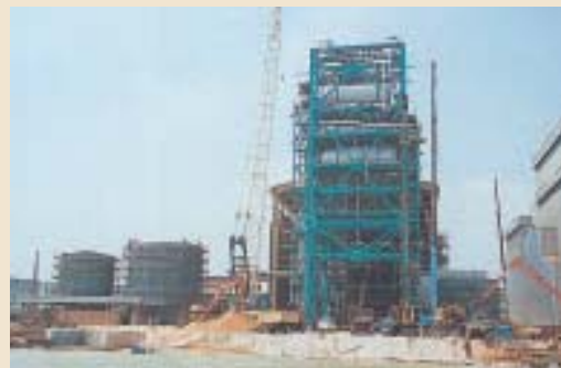
The PRAI combined-cycle power station under construction in Malaysia.
