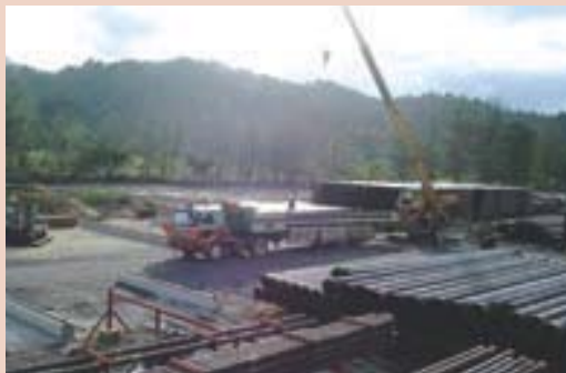
Steel pipe installation and inventory operation site in Malaysia.
