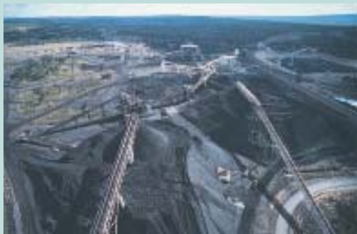
A plant on Oaky Creek coal mine.
