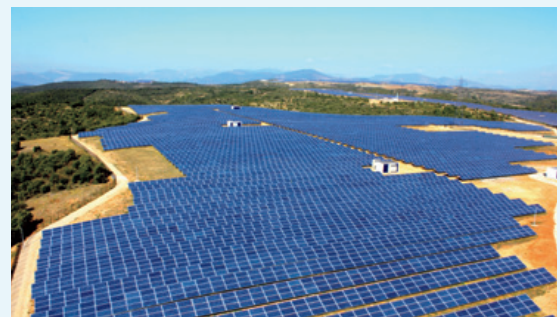
▶ Lavansol-1 solar power plant in France
