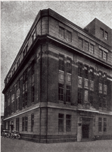
Sumitomo Building Annex where Nippon Kensetsu Sangyo's head office was located
