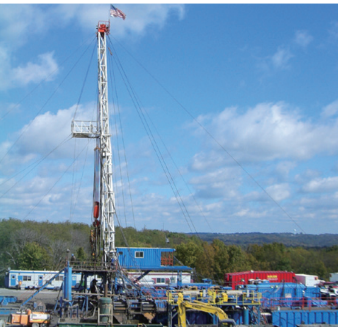
◀ A drilling rig in the Marcellus Shale Fields
