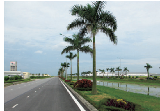
▶ Thang Long Industrial Park II in Vietnam
