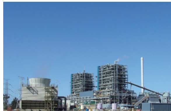
▲ The Bluewaters power station in Australia
