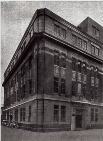
Sumitomo Building Annex where Nippon Engineering's head office was located
