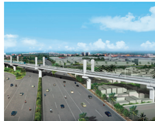
Completed image of Vietnam's first urban railway system
