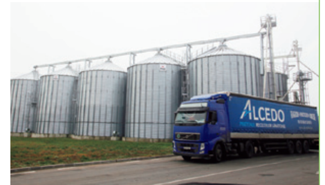
Alcedo's grain silos in Romania
