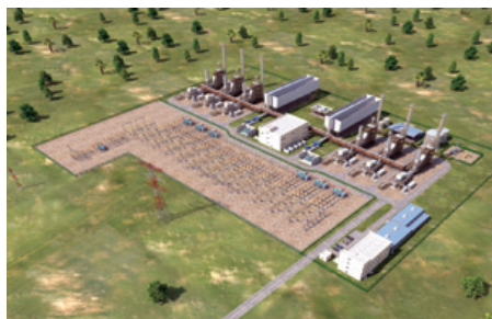
Image of completed Kinyerezi gas-fired combined-cycle thermal power plant (Tanzania)
