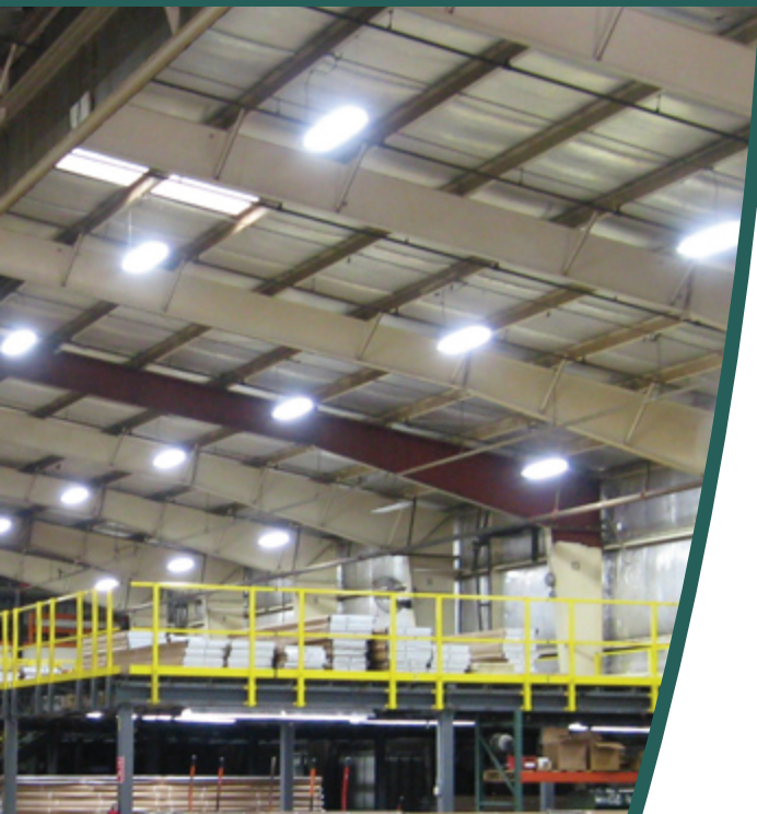
NEW WAREHOUSE LIGHTING
