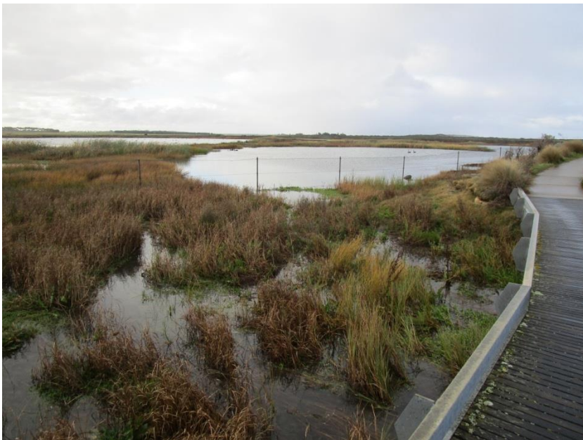
Stormwater overflowing into the wetlands at the south-western corner of the Karaaf.
