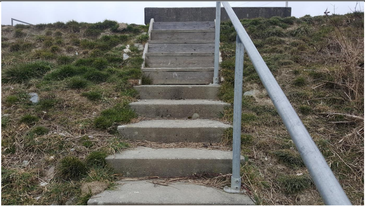
Photo 7 – South Stairs for Cloverdale Pump Station.
