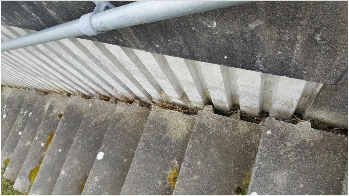
Photo 9 – North Stairs for Cloverdale Pump Station.
