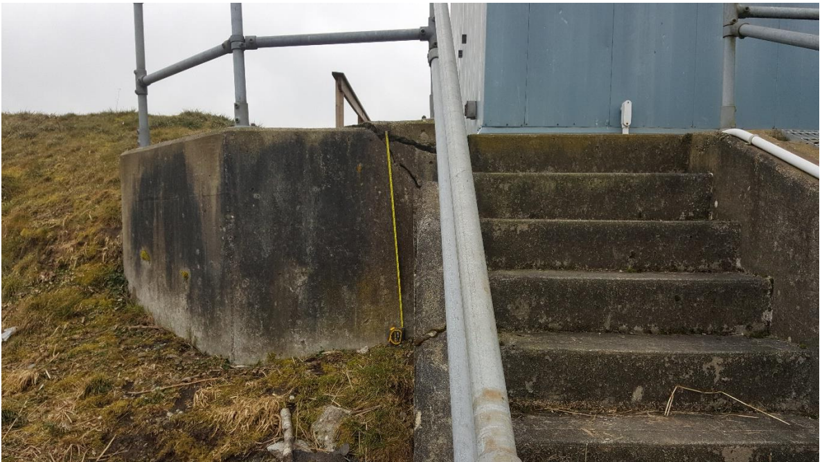
Photo 2 – Sloping of retaining wall for Erikson Pump Station.
