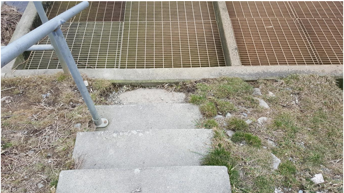
Photo 6 – Cloverdale pump station south stairs.
