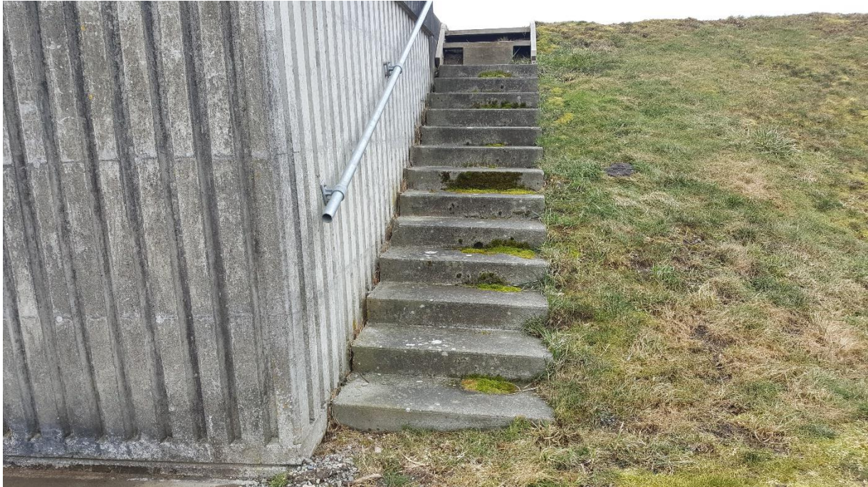
Photo 8 – North Stairs for Cloverdale Pump Station.
