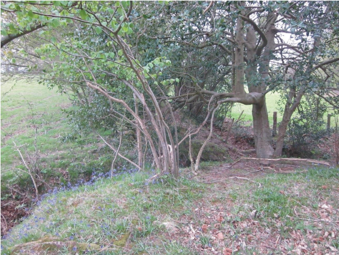
Figure 22 Modern drainage channel cutting earthworks at north-eastern side of Dry Hill Camp
