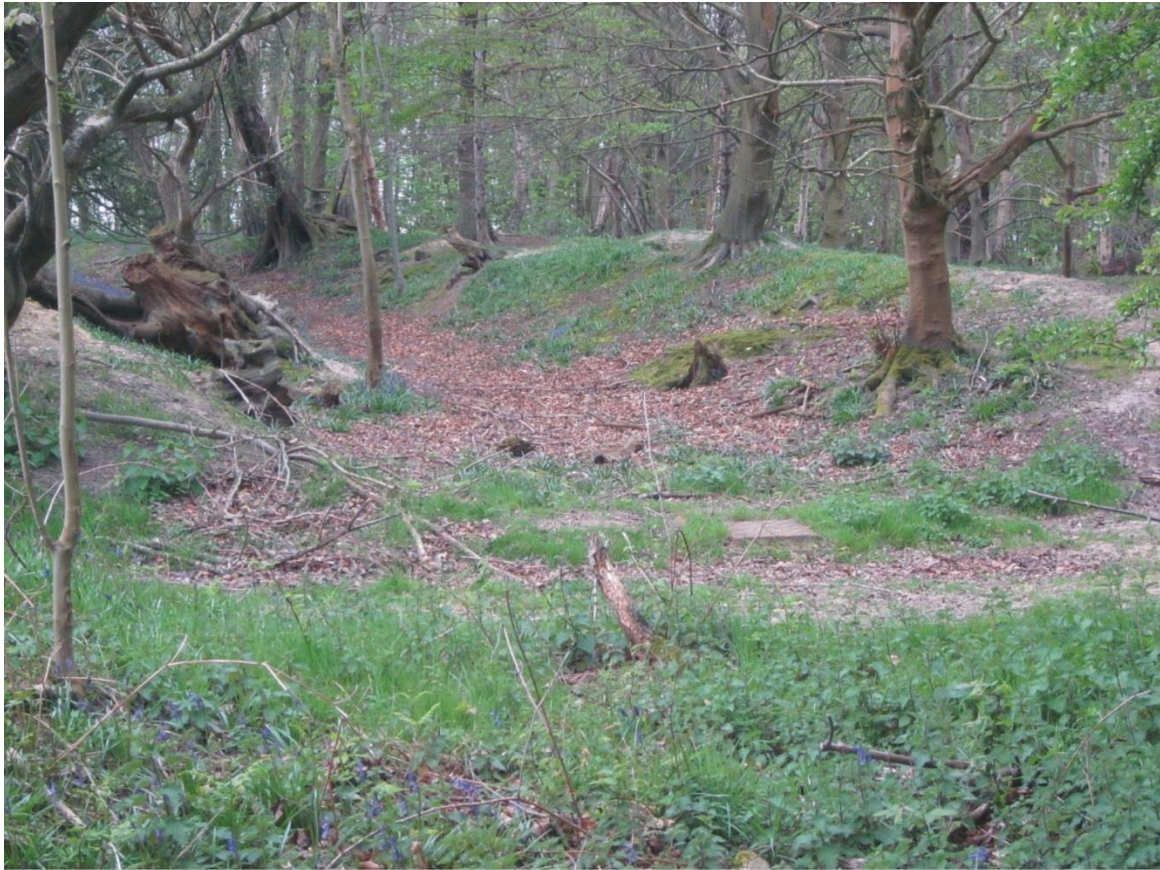
Figure 12 Cover for access to utilities pipe within 'Northern Entrance' at Dry Hill Camp
