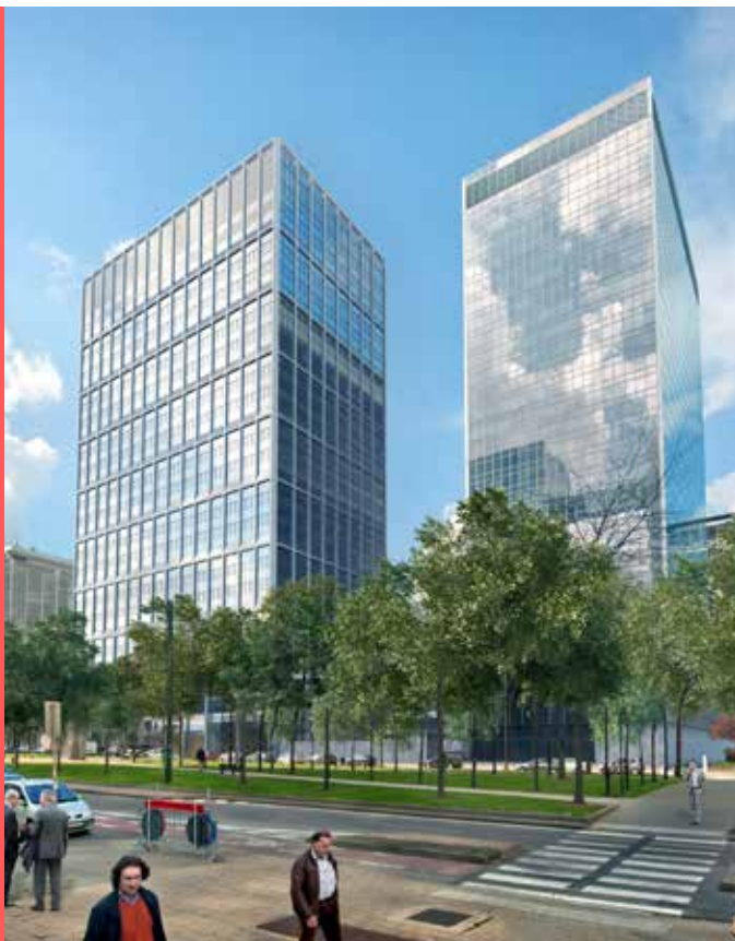
WTC IV, BRUSSELS NORTH AREA
