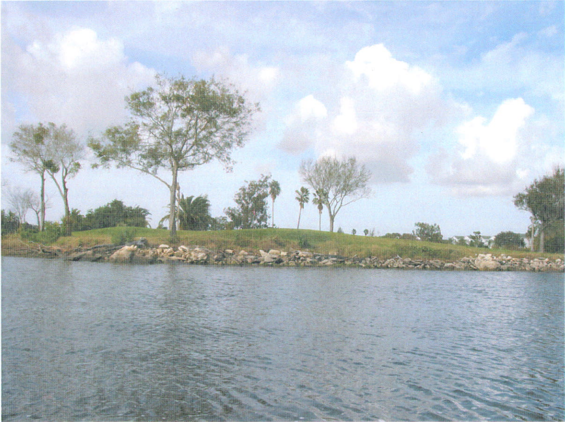
Figure 24: Golf course located on the northern bank at RK12 with rubble used to armor the shoreline.
