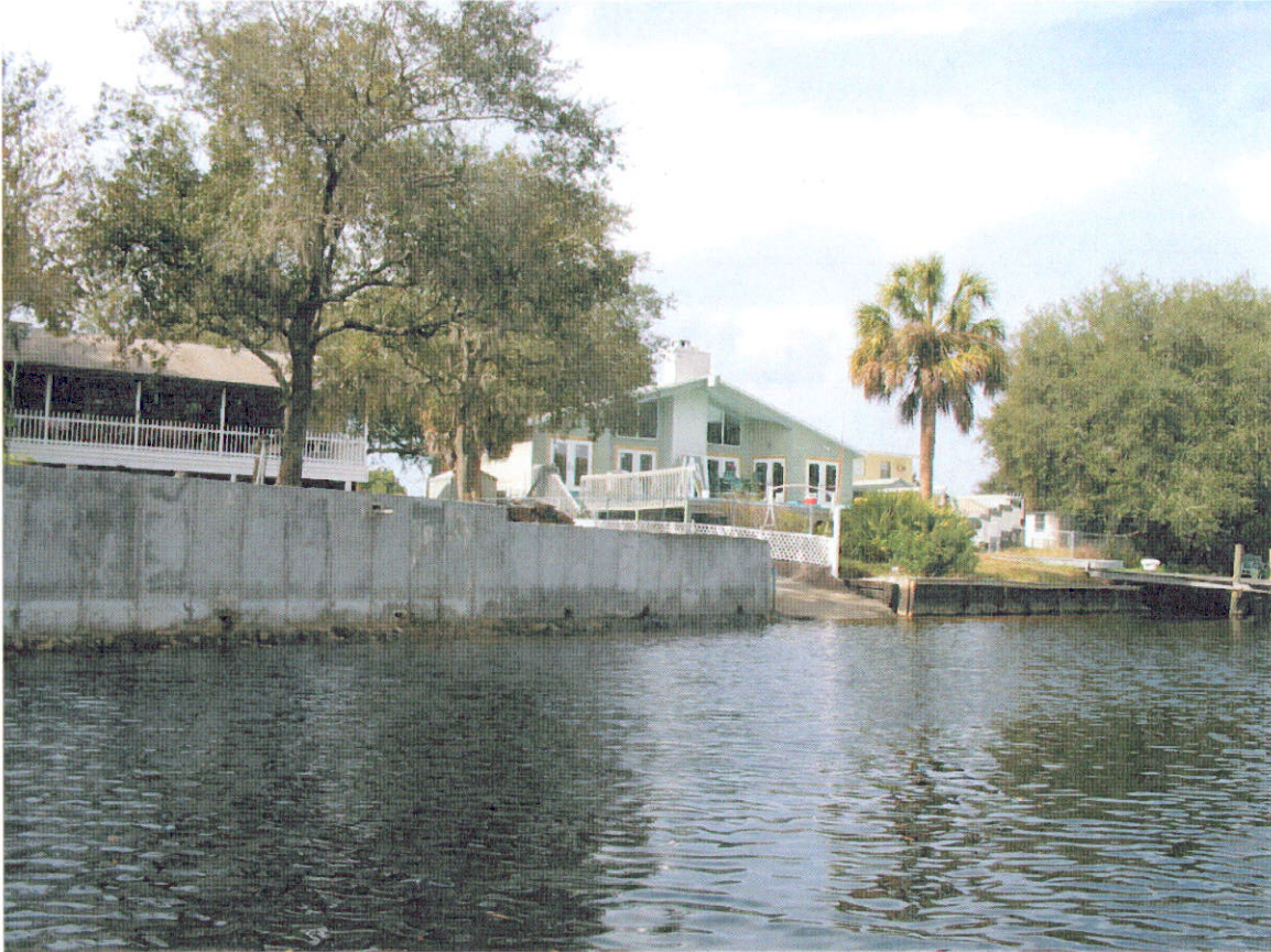
Figure 27: Two examples of concrete walls used to armor the shoreline.
