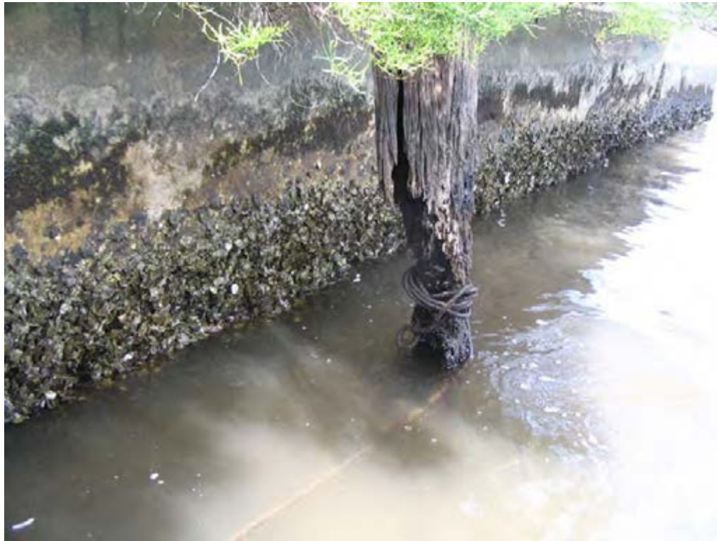
Figure 3.2-5. Oyster Colonization of Mud and Concrete Seawalls.
