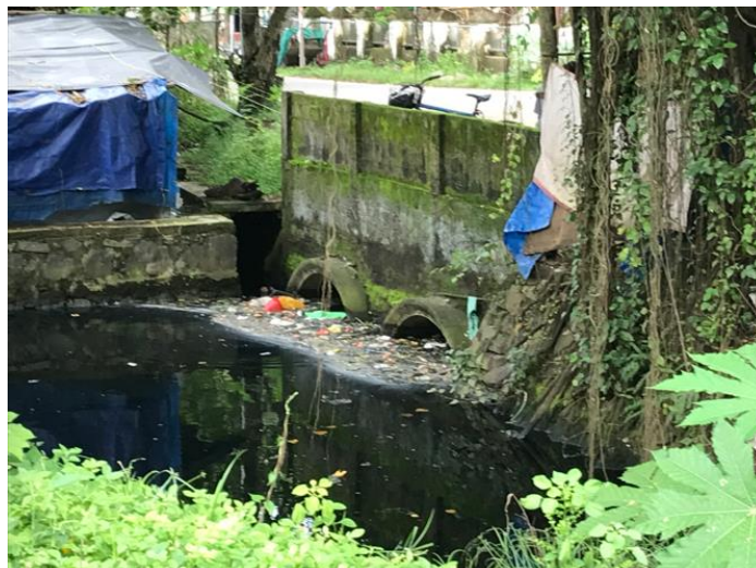
Figure 9. The bridge at Kochupally Road and the two culverts under the bridge.
