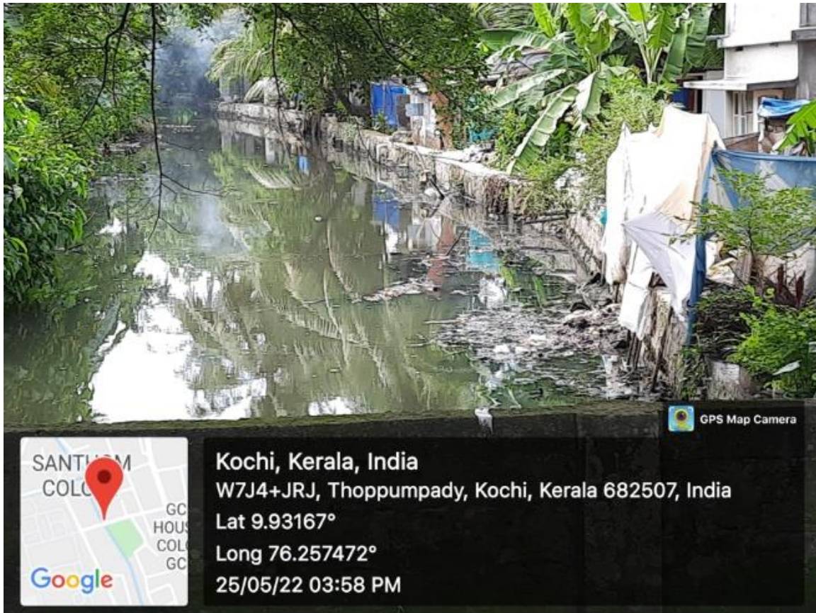
Garbage dumping area in the canal (Photo Credit: bechtel.org)
