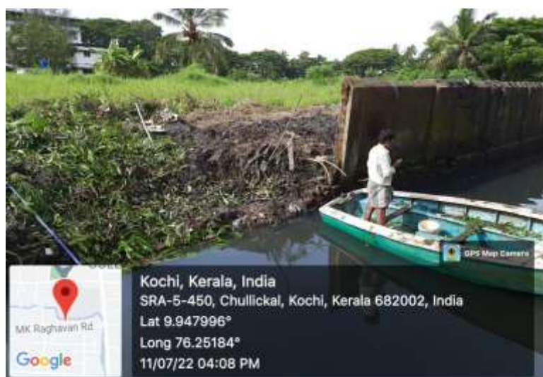
Figure 5-9 Canal cleaning activities
