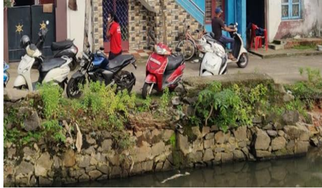
Figure 19: Relining of canals (Photo Credit: bechtel.org)
