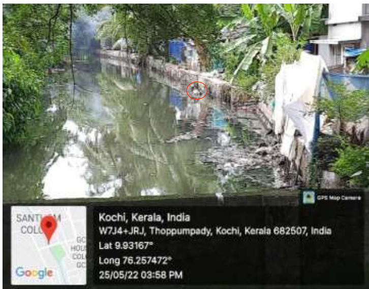
Figure 4-19: Direct discharge into the canal from toilet blocks
