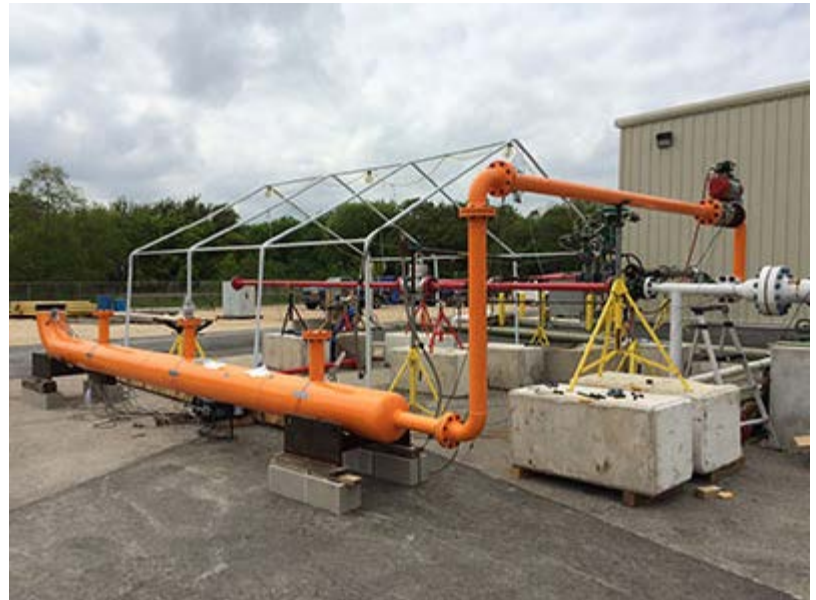
Figure 1: Installed test section (orange) in the parallel configuration.
