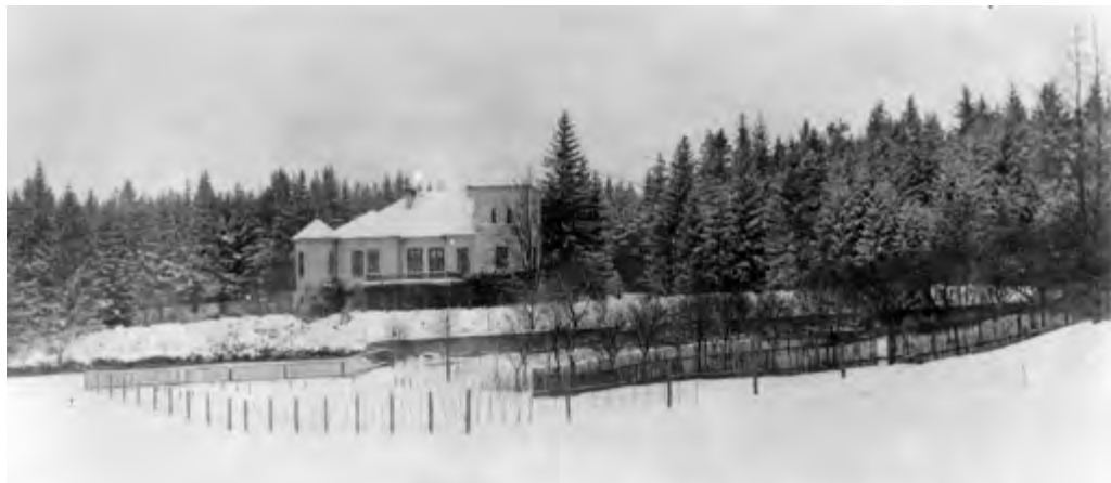
View of Nový Dvůr manor house (1910)
