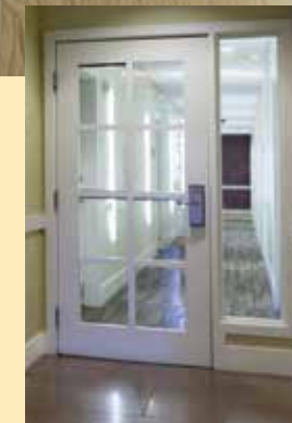
Fire rated 20 glass #8L in simulated divided lites
