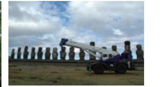
Moai Restoration Project
