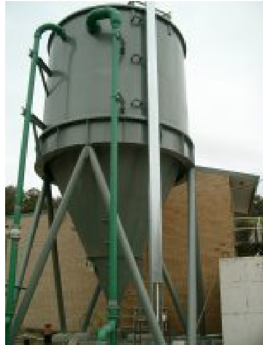
Figure 5: Deep cone thickener ( www.solid-liquid-separation.com ).
