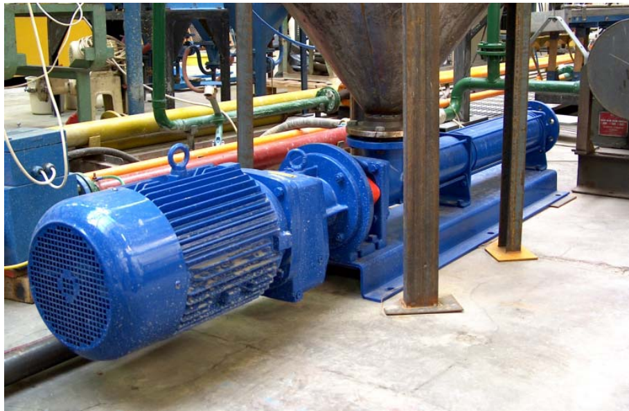
Figure 24: Mono type screw pump.
