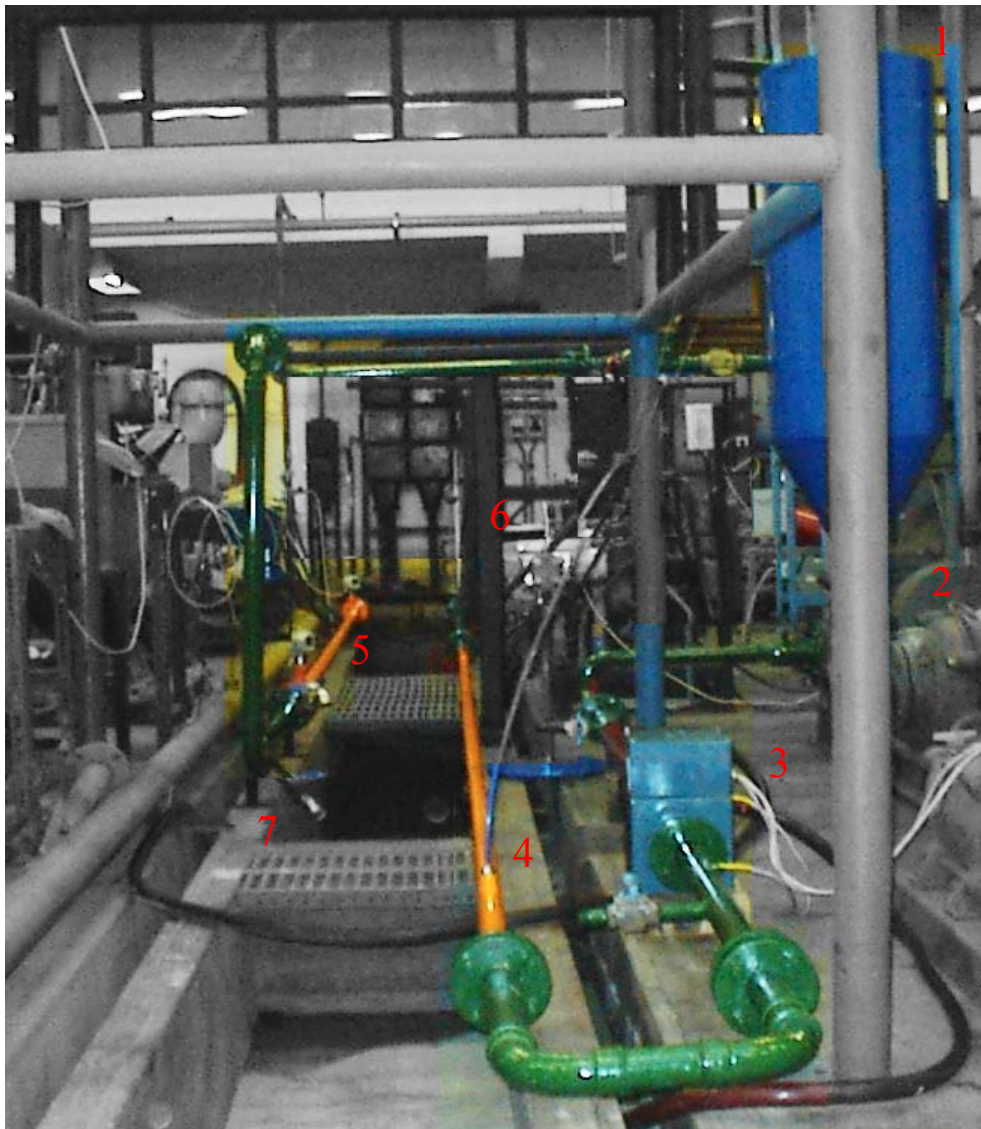
Figure 26: Picture of the hydraulic test system.
