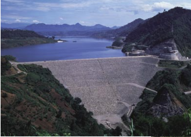
Cirata Hydroelectric Project, Indonesia
