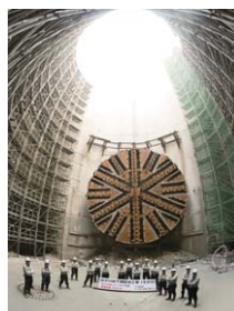
Shield machine for the Shirako River underground flood control reservoir
