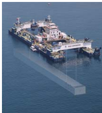
Bosphorus Straits Crossing Railway Immersion of tunnel element
