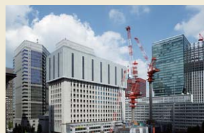
First case of application of the new demolition method "Tecorep System"
