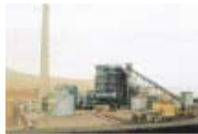
Coal-fired thermal power plant, Ilo, Peru
