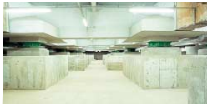
Yugawara Training Club: Eighth-floor Pillar where an antiseismic device was installed during the antiseismic retrofit construction work.
