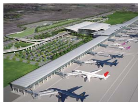
Noi Bai Airport, Vietnam
