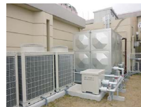
The energy efficient hot water heater EcoCute is installed in the caregiving facility "St. Joseph's Garden"
