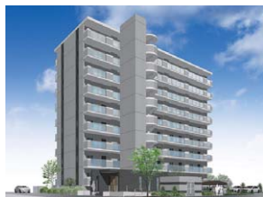
The ideal matching of PC construction method with the Hybrid TASS structural method
