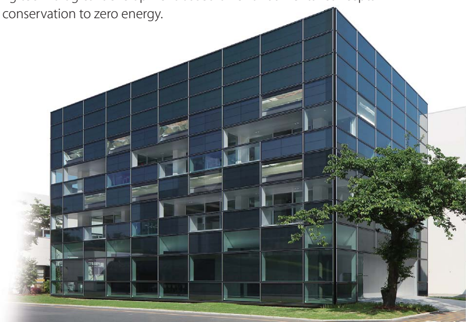
The ZEB Demonstration Building at the Technology Center. It was the first building in Japan to obtain the highest 5-star rank in the Building Energy-efficiency Labeling System (BELS)
