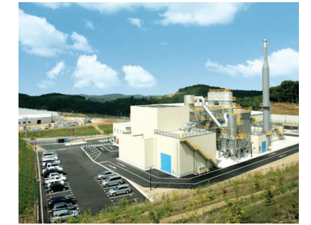
Plant that generates power from industrial waste and provides heat to a plantation
