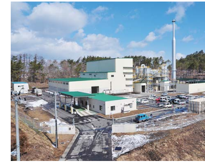
Industrial waste treatment plant
