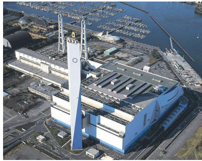
Energy from Waste plant
