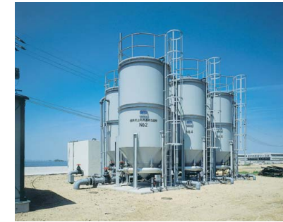
Upflow moving-bed filtration system
