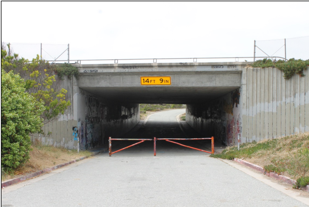
Photograph 9. SR 1 bridge over Divarty Street looking west. The Trail would begin on the west side of the bridge, follow the roadway to the point where it would transition to the grounds of the CSUMB campus.
