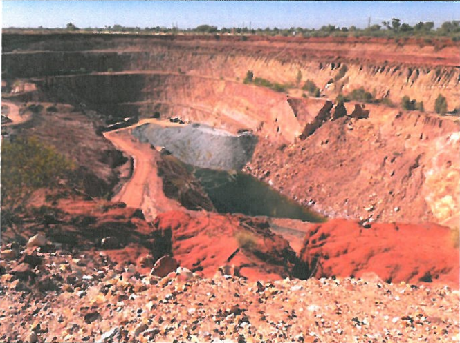
Photograph 15 – Pit 2, dewater pumped from this pit
