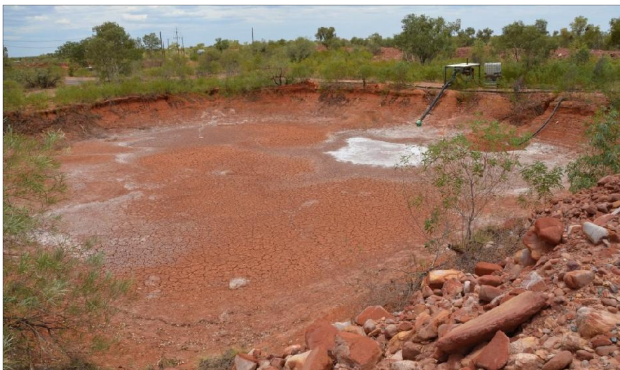
Plate 35: Surface water sump within the Coyote flood protection / abandonment bund
