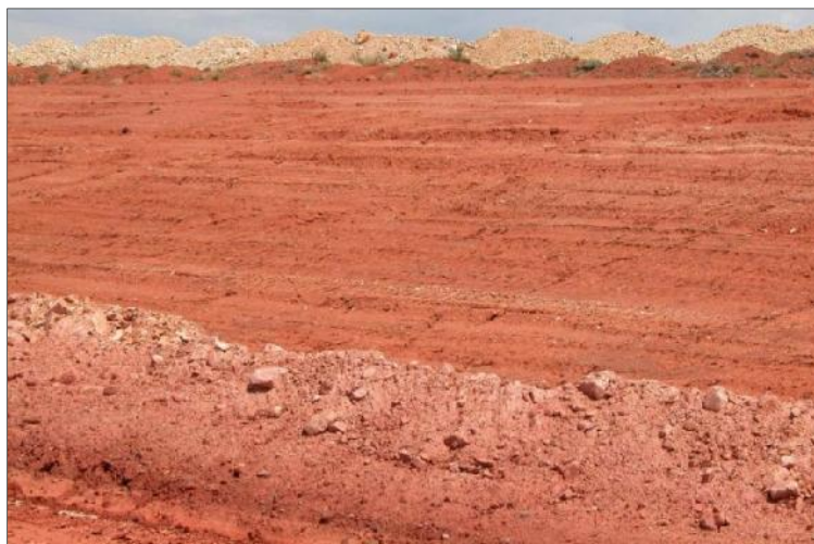
Plate 2: Coyote WRL following rehabilitation, February 2007 (TGNL 2008b)
