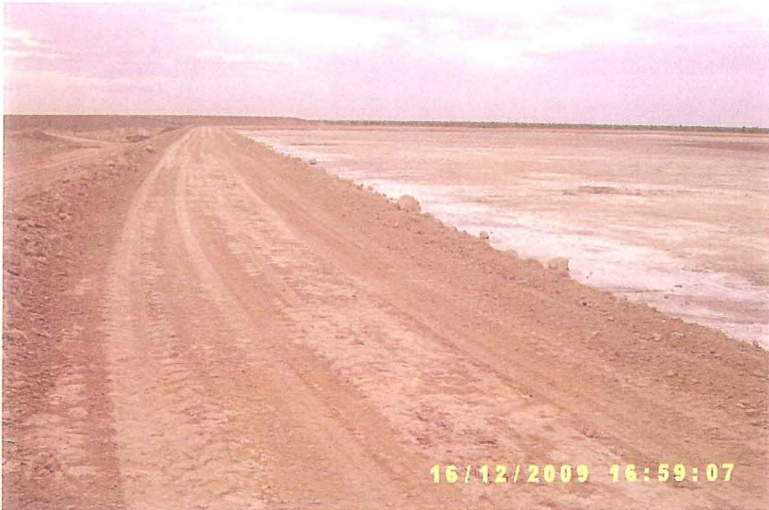
Photo 1: Tailings embankment lift at Tailings Storage Facility 1.
