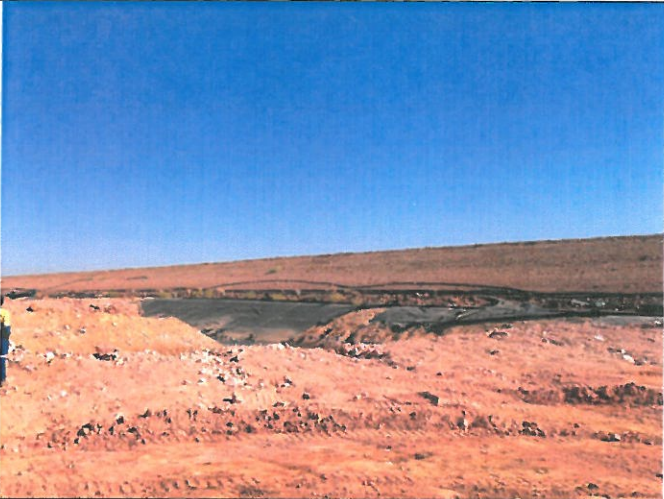
Photograph 9 – Inert Landfill adjacent TSF1
