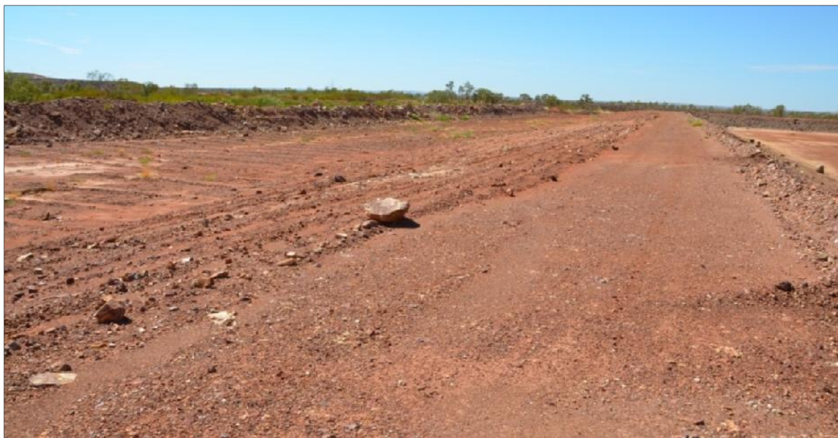
Plate 31: Bald Hill evaporation dam rehabilitation, looking south, November 2013
