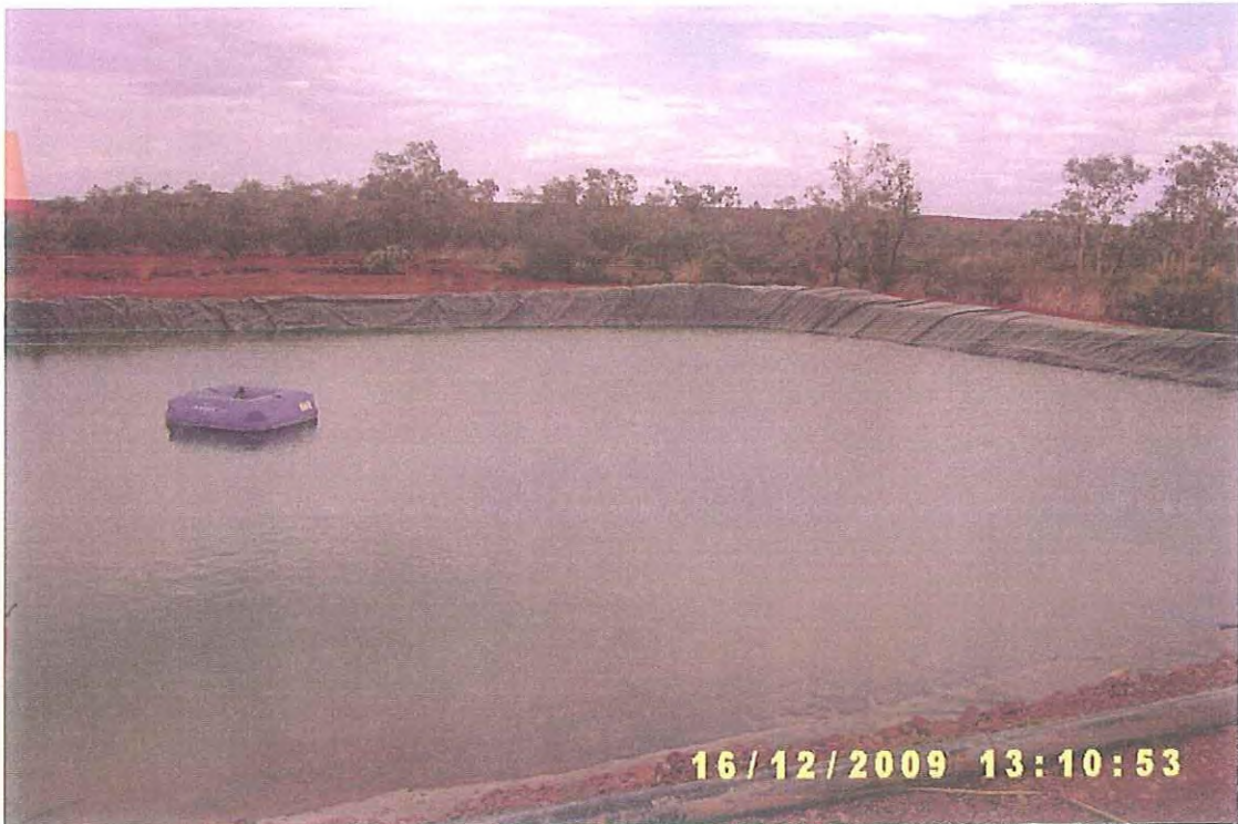
Photo 12: Turkeys Nest Dam at the Sandpiper/Kookaburra Project without Egress Matting.
