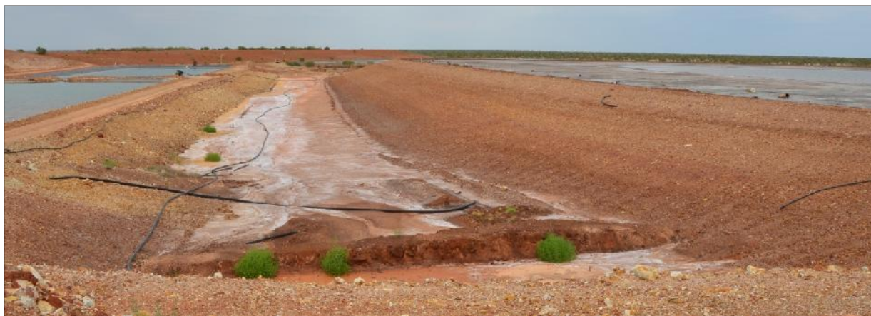
Plate 11: Seepage Trench between Cell 1 and 2, looking west along the southern embankment
