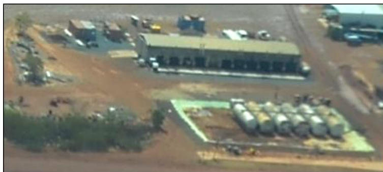
Plate 19: Power house, fuel storage and refueling bay, looking west, November 2013
