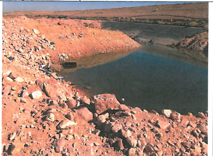
Photograph 10 – Vats for waste, located at edge of TSF1
