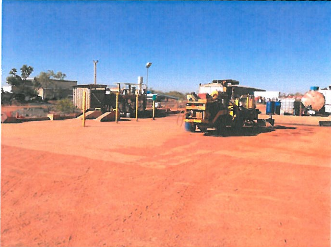
Photograph 3 – Wash down pad next to heavy vehicle workshop
