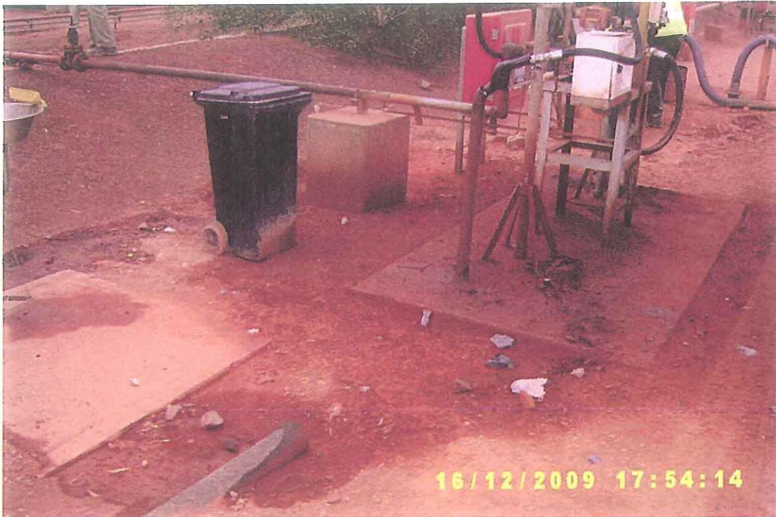
Photo 7: Hydrocarbon Contaminated Area Surrounding the Refuelling Area.
