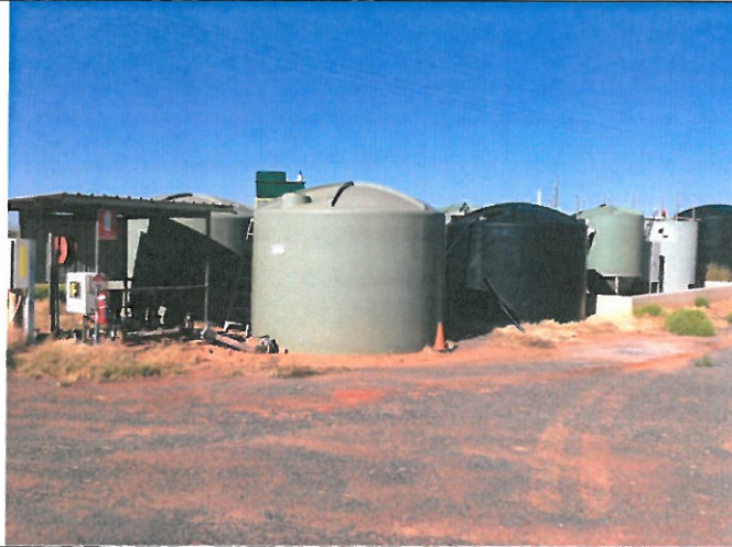
Photograph 1 – Sewerage Facility, end water to TSF
