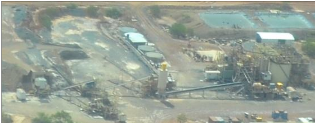
Plate 17: Coyote Process Plant, looking west, November 2013
