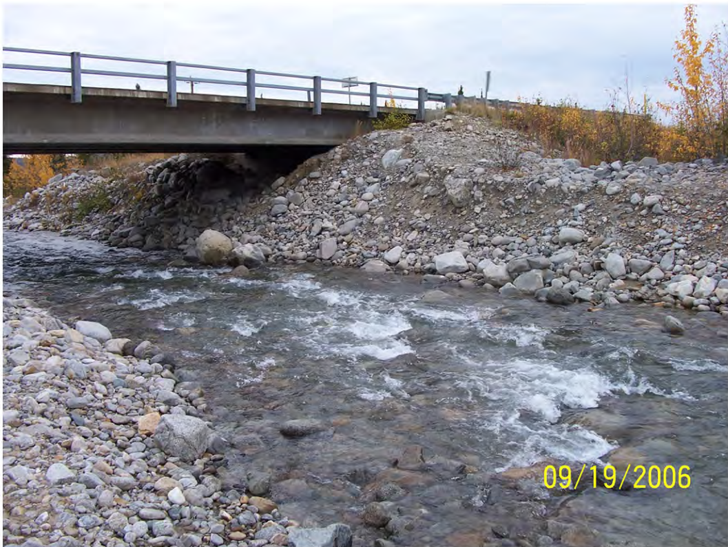
Above Photo: Alaska Highway crossing over Yerrick Creek
